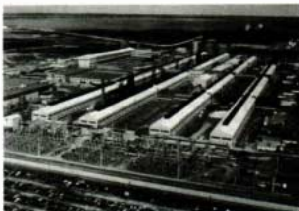
Figure 1. An aluminum plant. Each of the electrolytic cells is arranged in electrical series in "potlines," and the plant may align several potlines. Each cell provides electrochemical resistance.
